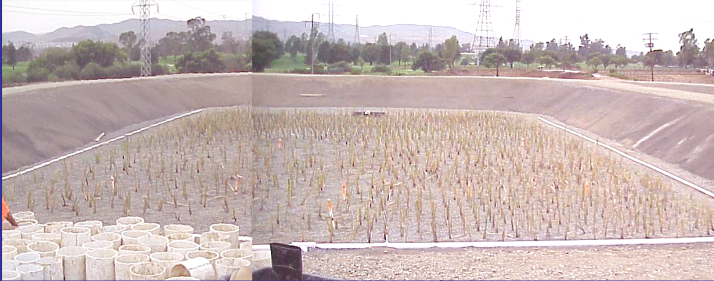
Side-loading constructed wetland
