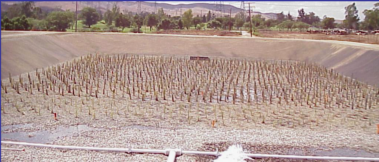
Front-loading constructed wetland
