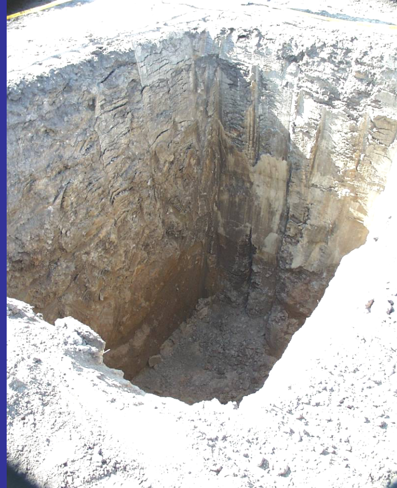
Excavation of the facultative digestion pit (5 m deep)
